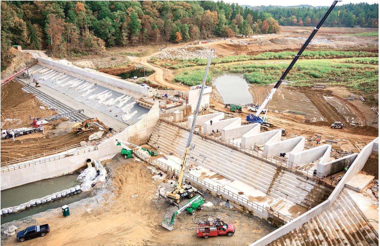
The rehabilitated Lake Williams Dam features a labyrinth weir and spillway. Once full, the reservoir will include 'turtle island' and aquatic habitat features.
