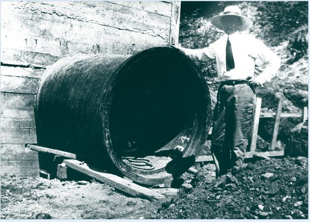
Above: Lake Williams spillway under construction in 1911. Below: A foreman poses at the 48" diameter outlet valve during construction in 1911.
