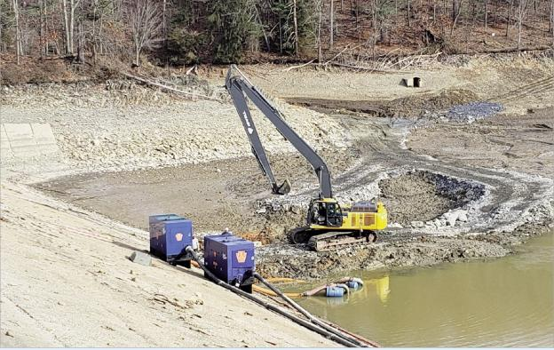
In 2018, construction began on several projects at Lake Williams. The first project is the installation of a valve on the 48" outlet pipe passing through the dam (shown in these pictures). Lake Williams was drained down for this portion of the work. When this work is completed in 2019, the lake will be allowed to refill and then the spillway will be replaced with new concrete, and then a roller compacted concrete armoring project will take place on the downstream face of the dam.
