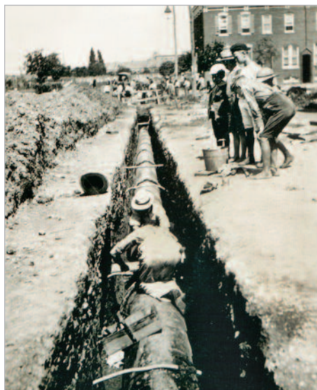
Plumber wiping joint where service was cut so as to make room for 20" supply main. August 28, 1898.
