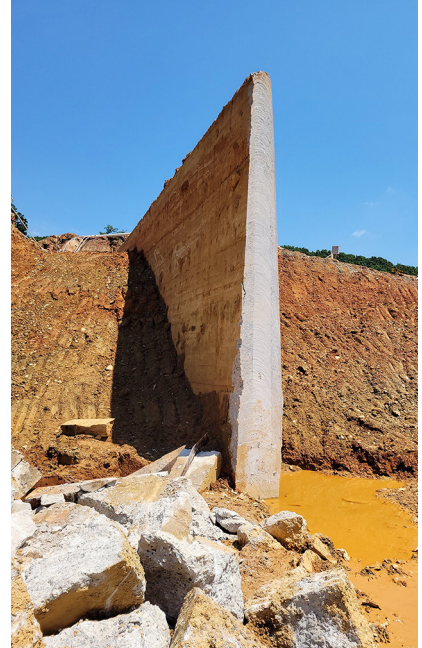
1912 concrete core wall
